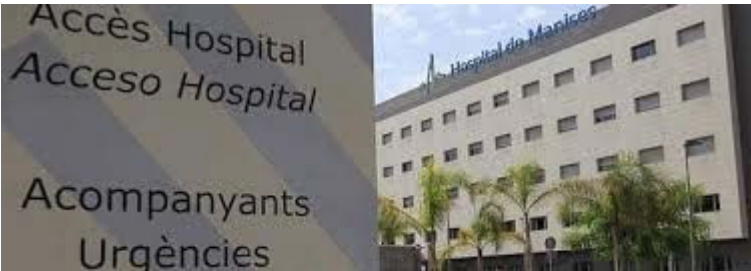
The Sanitas 35 year contract to manage the whole population of the Manises district of Valencia
